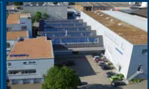
Plant Aadorf, Switzerland GRESSEL AG Schützenstr. 25 CH-8355 Aadorf Tel. +41-52-368-16-16 Fax +41-52-368-16-17
